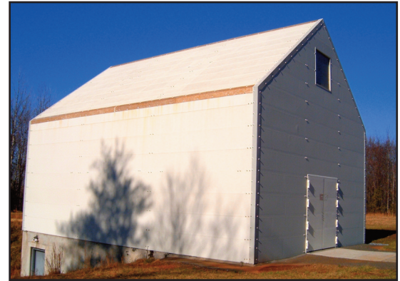
The lab consists of a 30 x 34-foot non-metallic building invisible to electro-magnetic emissions.
